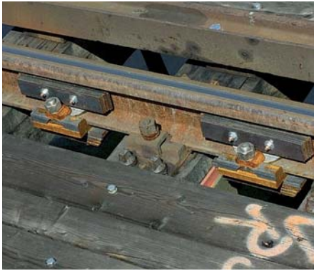
Abb. 3: System Schrey & Veit (Schichtabsorber)
